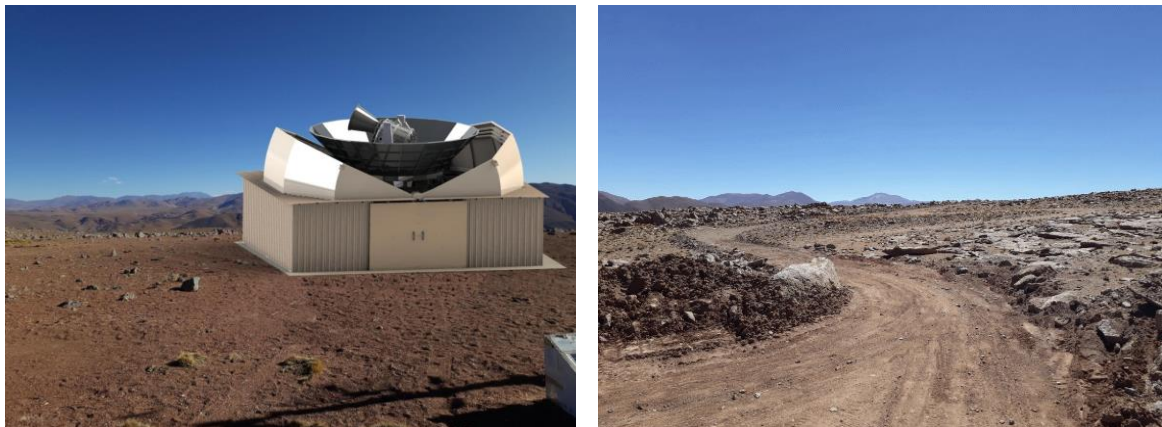
Figure 1: Rendering of the shelter with the opened dome, the groundshield and the instrument in its center (left). Access road to the QUBIC site (right).
